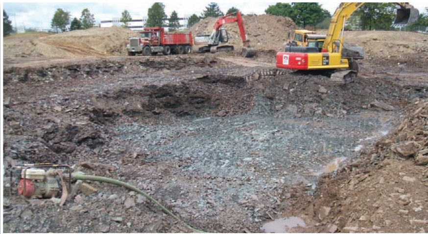
Phthalate excavation area.
