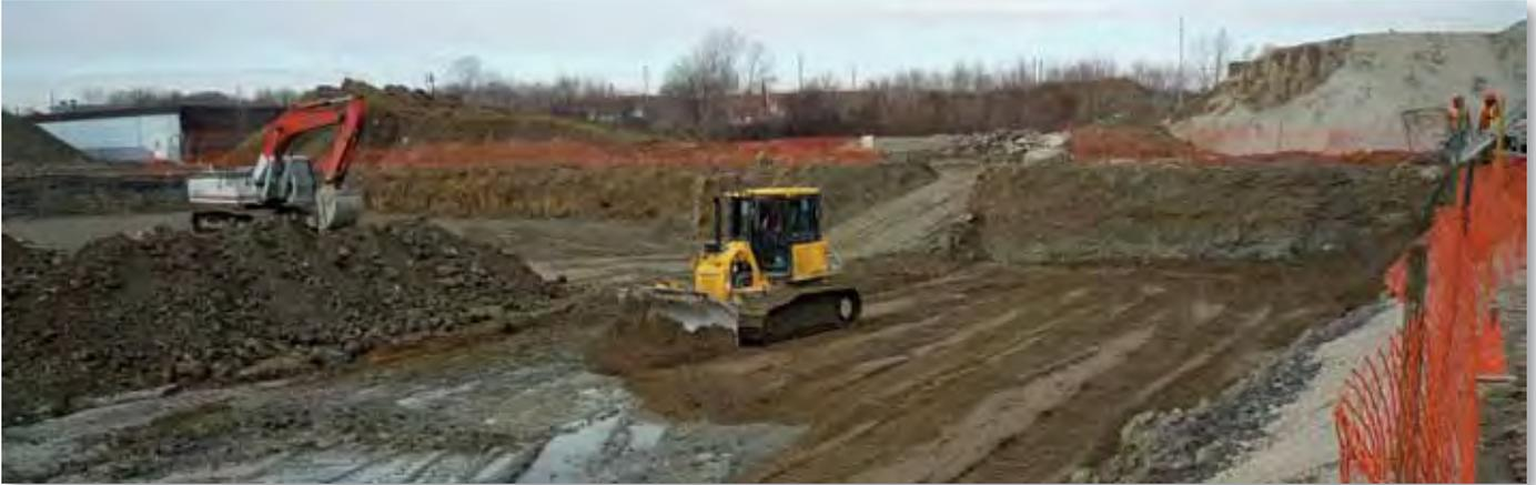
*Excavating the site: soil was reused and groundwater was treated with the ZVI-clay technology.*
