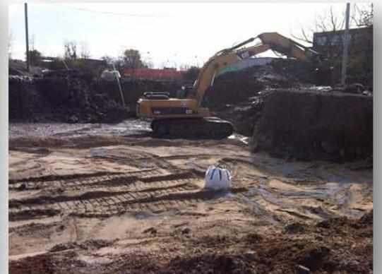
**ZVI AMENDMENT** | Treated soils were backfilled with Zero-Valent Iron (ZVI)/sand layers in excavated areas. This technology received the generous support of Sustainable Development Technology Canada's (SDTC) Tech Fund.
