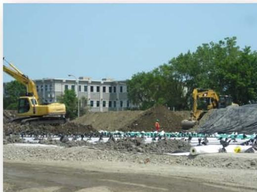
**BIOREMEDIATION** | 14,500 m<sup>3</sup> of soils impacted by various organic parameters were treated using bio-remediation. Treated soils will be re-used on site.
