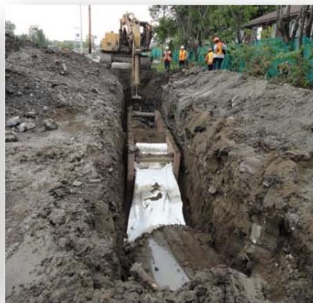
**PERMEABLE REACTIVE BARRIER** | A PRB was installed around a portion of the property boundary to mitigate any migration of cVOC-impacted ground water.
